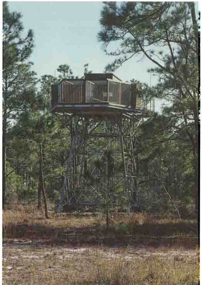
Figure 6. Hacking towers, this one on Horn Island, Mississippi, are placed in isolated patches of vacant habitat in an effort to reconnect the relict populations remaining in the Southeast. Cages containing artificial nests surround a central observation room from which the birds, unaware of their human caretakers, can be fed and observed. (Photograph by T. Simons.)
